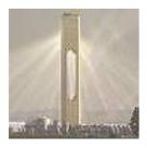
Solucar 600-mirror Solar Tower in Seville Spain is the first commercial concentrator station in Europe. It focuses Sunlight onto water pipes at the top of a 40-storey concrete tower, which drives a turbine to generate 11 megawatts of electricity. Thousands more mirrors will be added to further boost the output. Added details: http://www.solucar.es/
